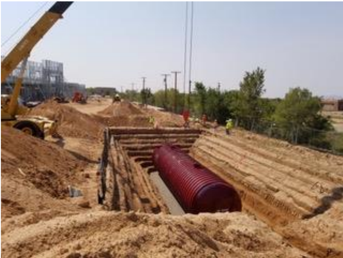
Figure 6. Installation of a 40,000-gallon cistern in 2018 at Milagro for irrigation purposes. Photo courtesy of Reese Baker.
