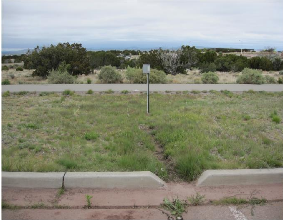
Figure 3. Curb cut without a rain garden (i.e. Control).
