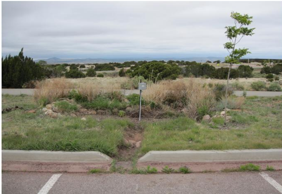
Figure 4. Curb cut with a rain garden (i.e. Treatment).
